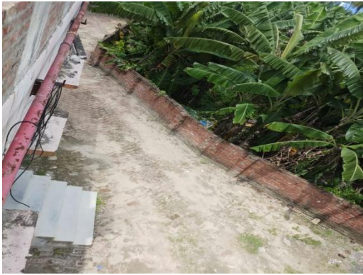
A VIEW OF THE BOUNDARY WALL
